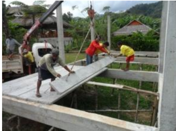
New multi-purpose building under construction
